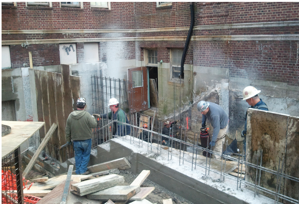
Work underway at Presentation School, Brighton MA
